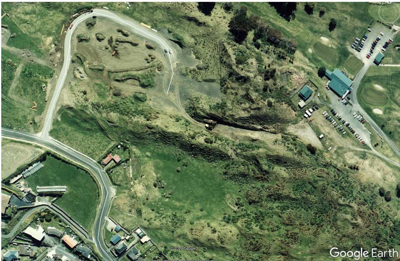
Photograph 4 : Aerial view from 2005 during construction of Golf Vue development. (from Google Earth)
