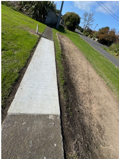
Footpath (fixed sections, not whole path) beside steep open drain. Look at the high lip.
