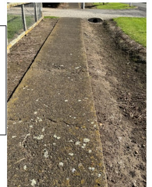
Footpath has a huge high lip, that then falls down into an open drain
