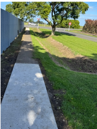
Footpath (fixed sections, not whole path) beside steep open drain. Look at the high lip.
