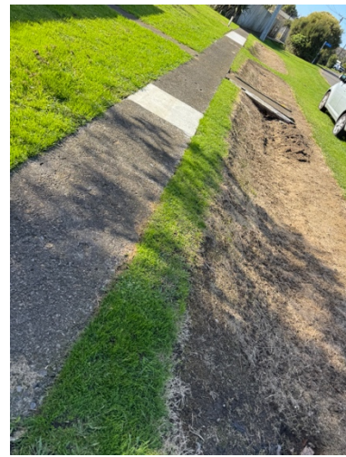
Narrow footpath right beside open drains, when it rains these become full of water.
