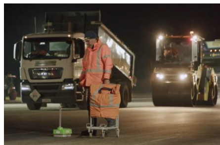
Testing the new surface
