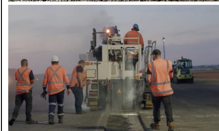
Milling off the old surface
