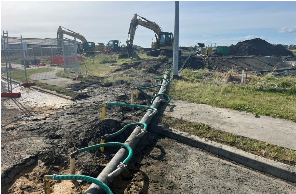
Figure 2 : Installation of dewatering spears in Fitzherbert Ave.
