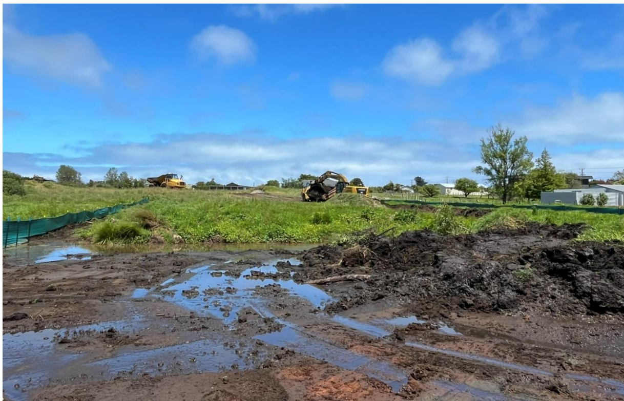
Figure 8 : Groundwater / perched water at ground surface at Fox Road end.
