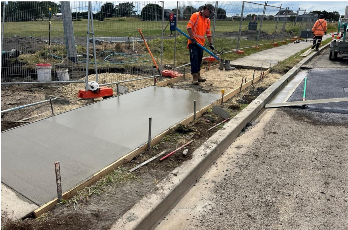
Figure 10 : Pouring concrete footpath on Fitzherbert Ave.
