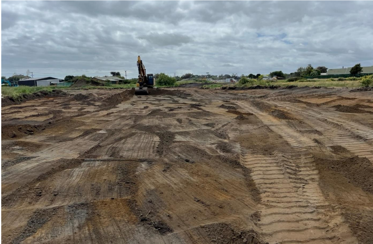
Figure 9 : Cut to fill (stockpile temporarily) started at Fitzherbert Ave end of site.
