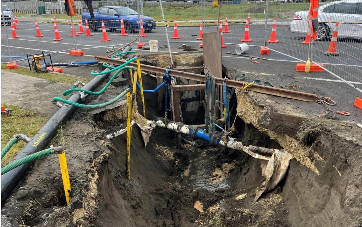
Figure 5 : Construction of sewer connection to existing manhole. Existing services supported within the excavation.
