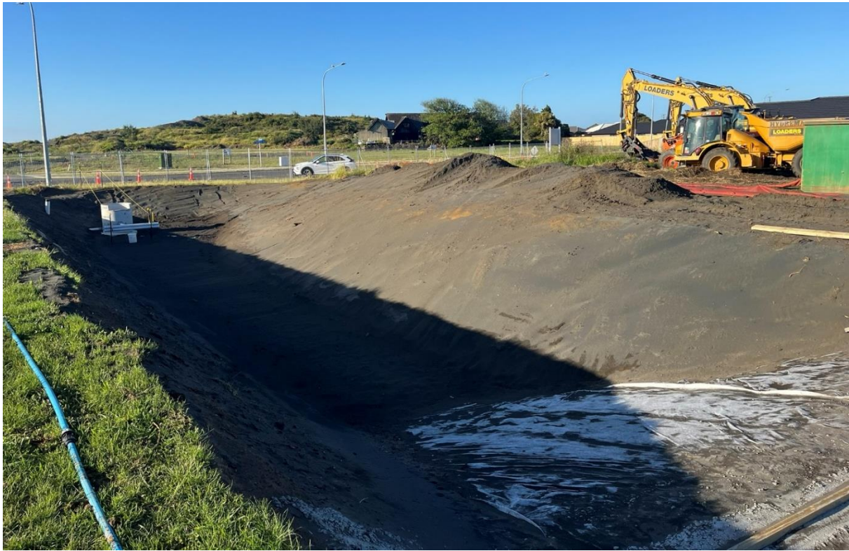
Figure 1 : Construction of the SRP level spreader, primary spillway and decant.
