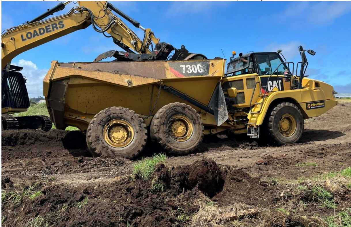
Figure 7 : Soft ground and groundwater encountered at Fox Road end of site. Dumper sinking in soft ground.
