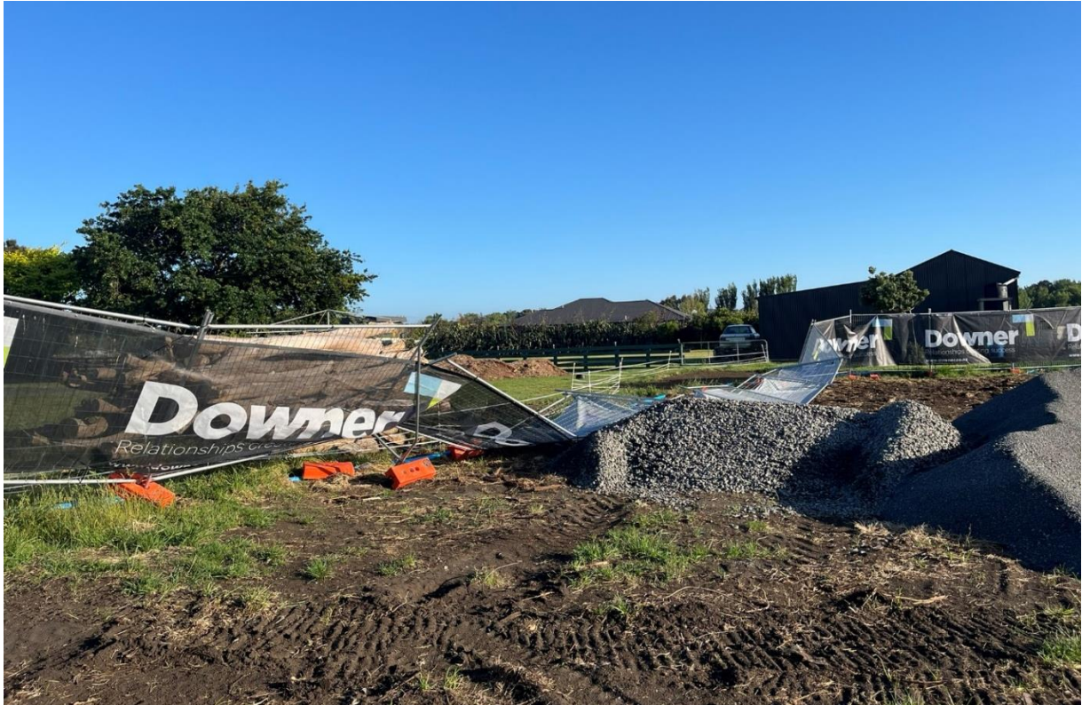
Figure 3 : Wind damage to 130 Mosston road fencing.
