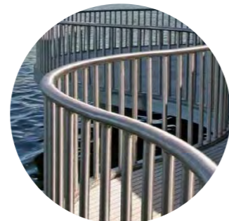
Steel handrail to follow shape of lookout
