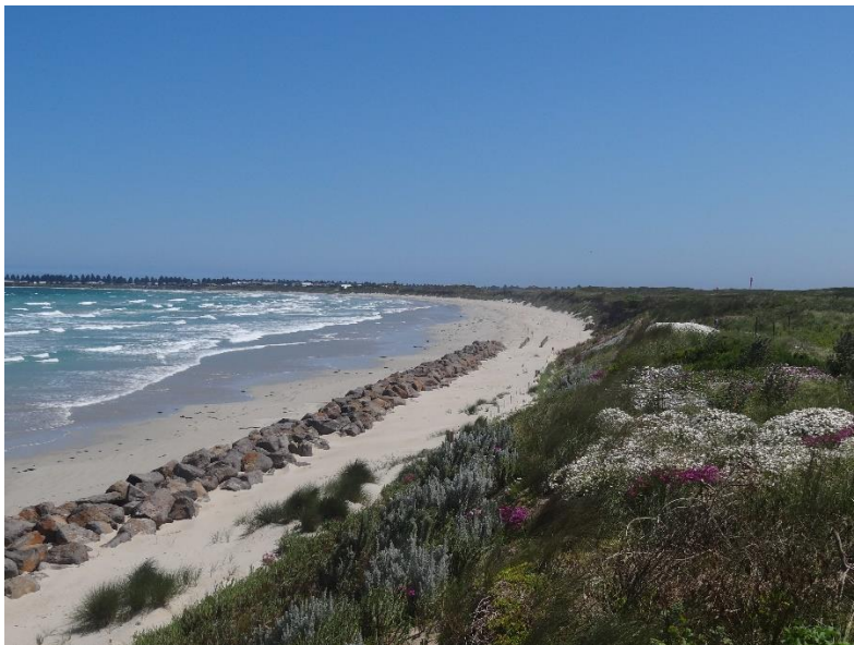
Photograph 3.8: Example of a rock sill on an open coast beach at Port Fairy, Vic (source: T+T)
