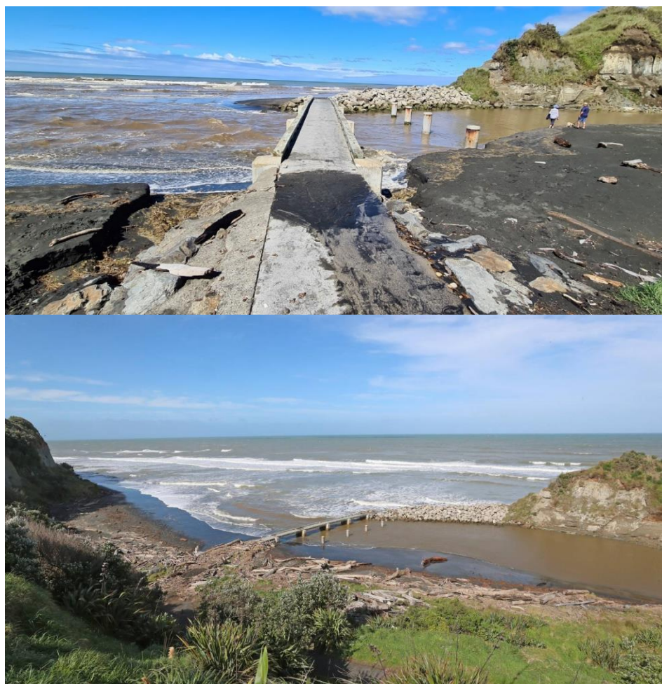
Photograph 2.3: Archers Bridiget crossing the Kai Iwi Stream mouth with a small rock abutment on the landward side and a low rock breakwater linking the seaward end of the bridge with the cliff (source: Top - WDC, 2022, Lower – Whanganui Chronicle Dec 2021)
