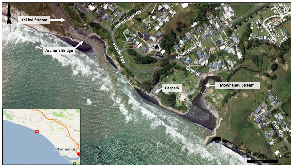
Figure 2.1: Overview of the site at Kai Iwi/Mowhanau Beach overlaid on the 2022 aerial photograph (sourced from LINZ)
