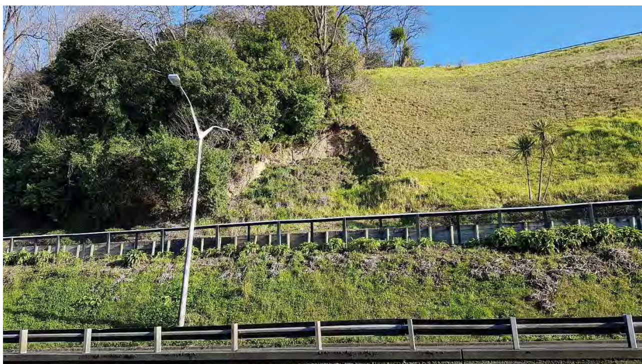
Illustration 5-3 : Landslide on steep slope
