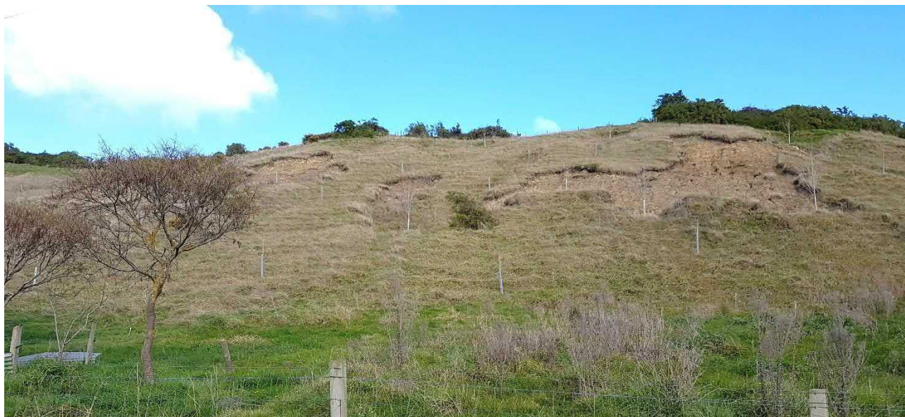
Illustration 5-2 : Shallow landslides in surficial topsoil/regolith
