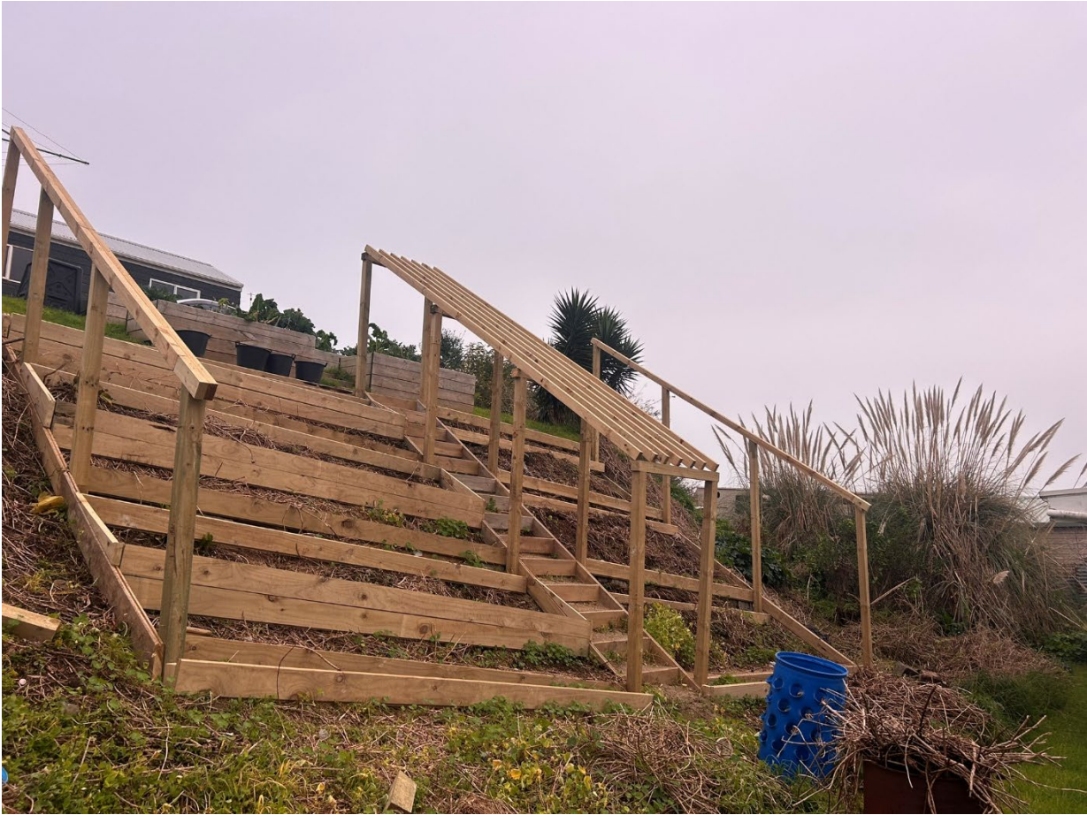
FIGURE 8: 68 CORNFOOT STREET (FACING WEST)
