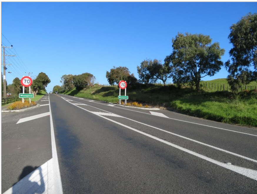
Photo -4 State Highway 3 opposite Bristol Property
