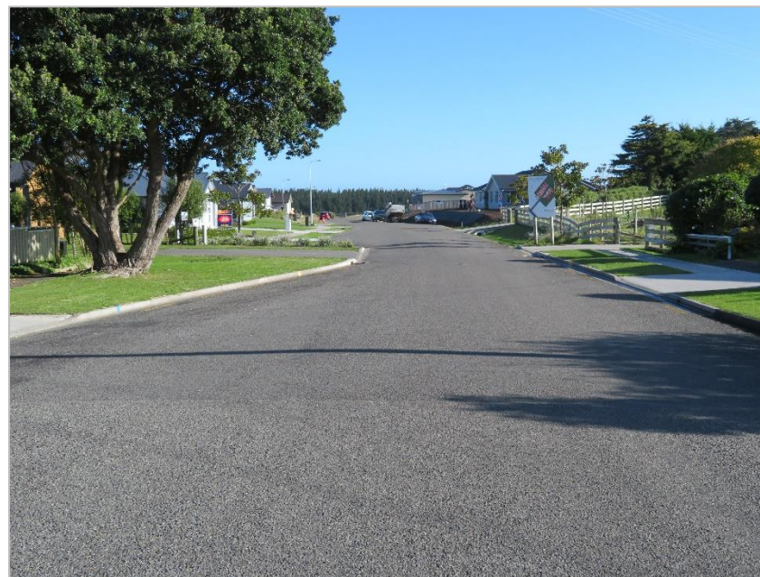
Photo 1 – Tirimoana Place Residential Development Stage One
