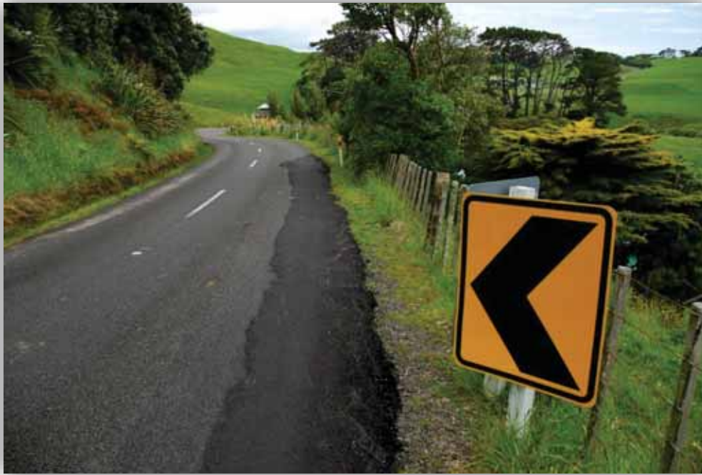
Illustration 3 Area of repaired cracking/settlement in the road pavement and shoulder, with tilted fence indicating soil creep below Handley Road, Mowhanau.
