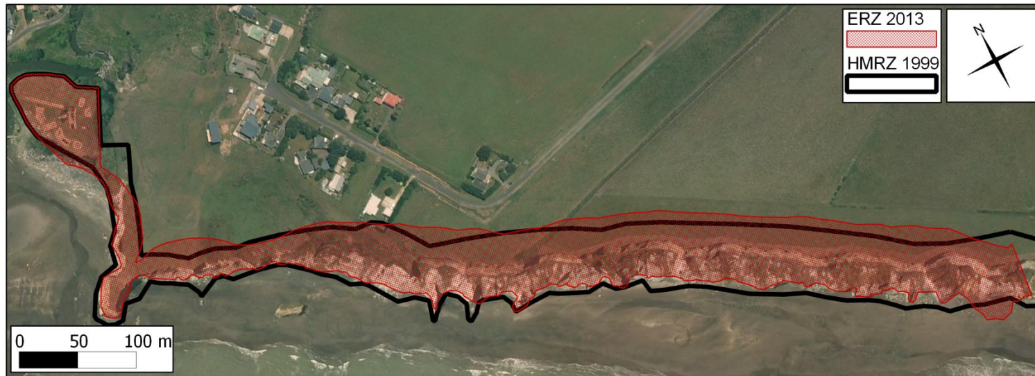
Figure 3.9. Mowhanau Cliff and Southeast Cliff section ERZ
