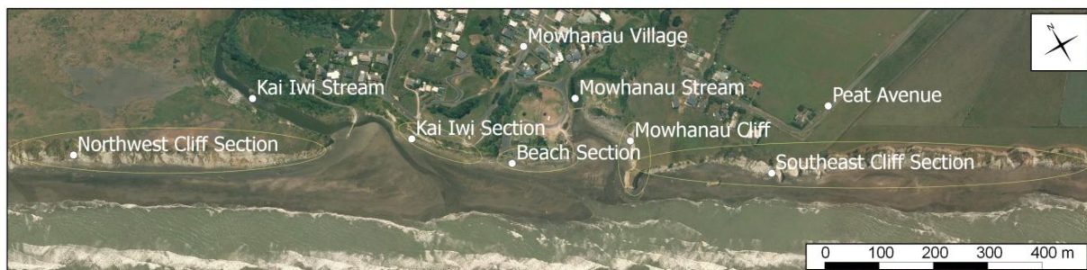
Figure 2.1. Ortho-rectified 2011 image of Mowhanau Village with prominent features and cliff line sections annotated
