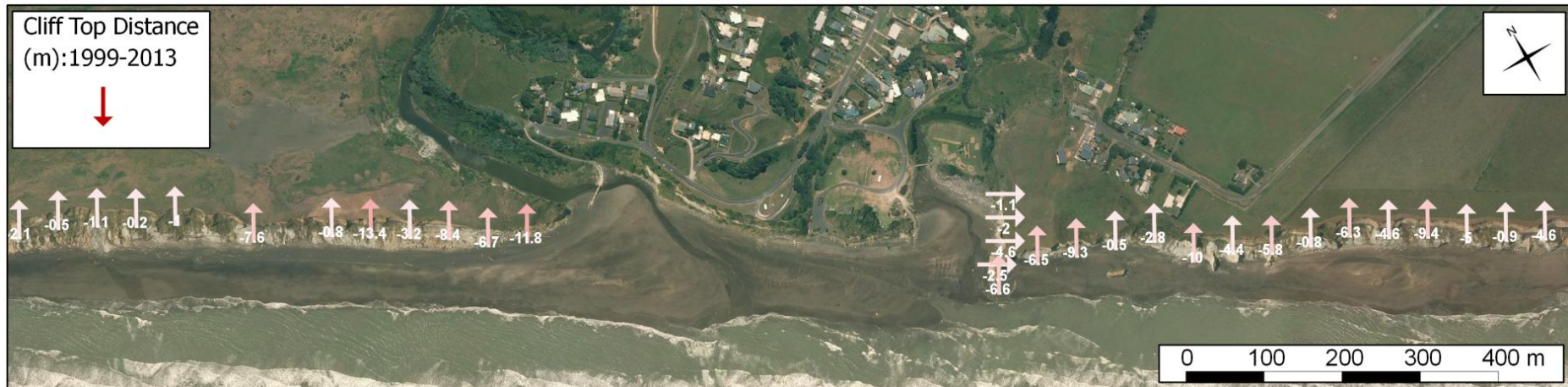
Figure 4.1. Cliff top erosion rates for the 1999 to 2013 period.
