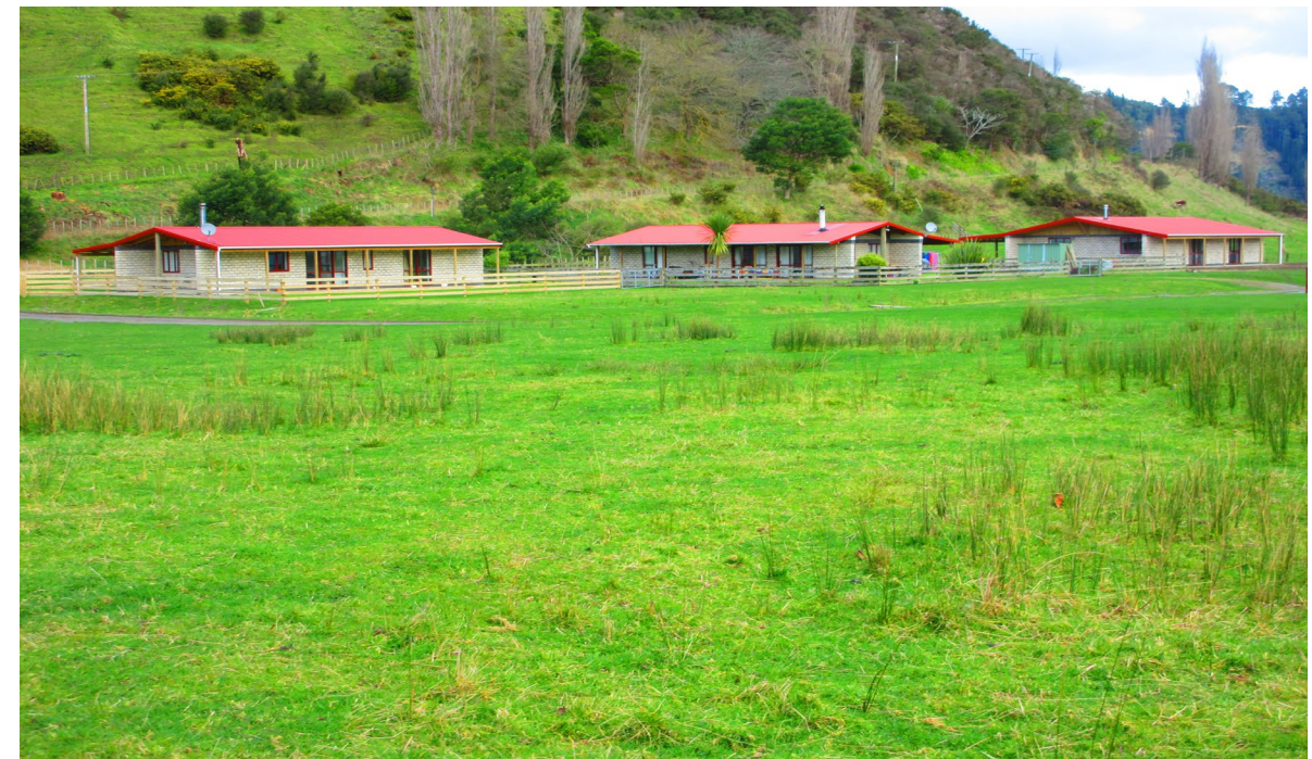
Figure 16 Papakāinga (whare kōhatu housing) at Pungarehu
