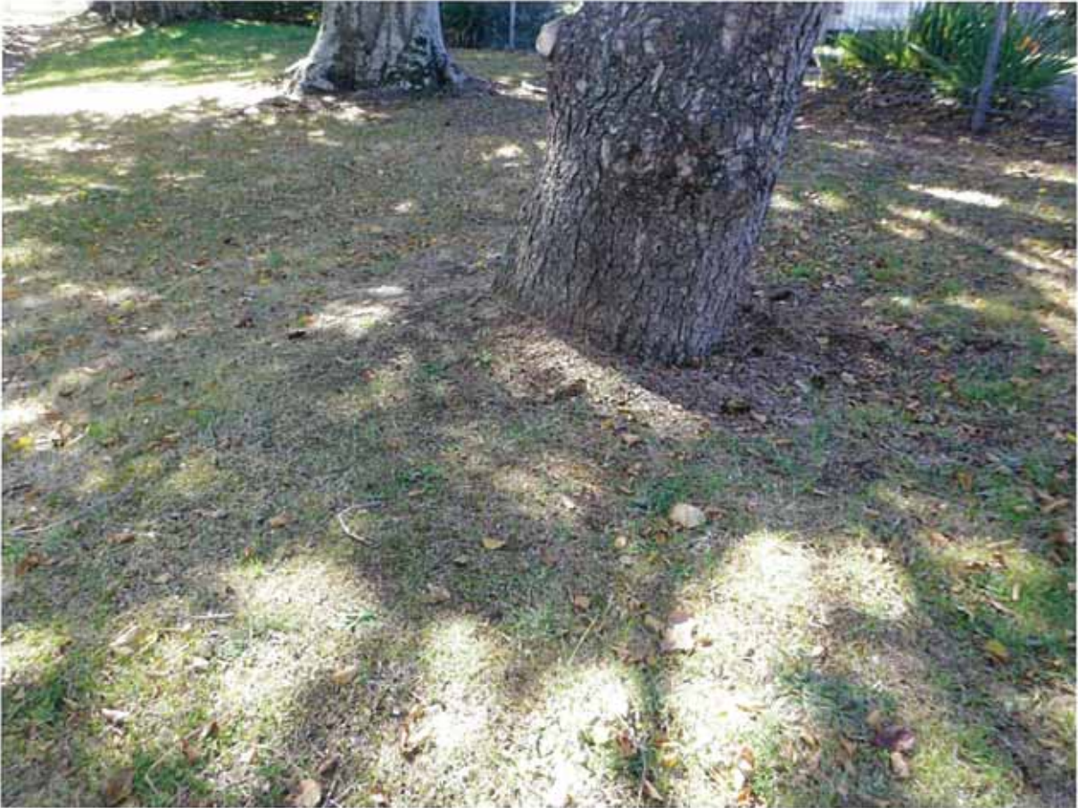
Tree 5/5 showing depression (right of trunk) and rise (left of trunk) which indicate a past partial root plate failure.
