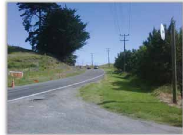
Figure 17 – Poor sight distances evident along Mosston Road
