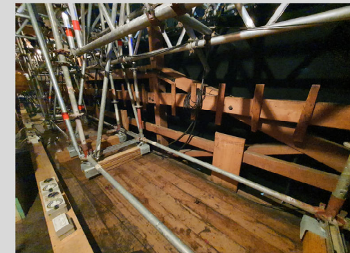
From left to right: Stage house roof structure / Unprotected wiring / Stage house wall timber structure (no lining or insulation) / House curtain rigging / Stage drapes / Fly floor railing & rigging scaffolding
