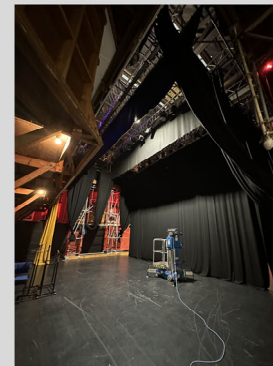
From left to right: Stage house roof structure / Unprotected wiring / Stage house wall timber structure (no lining or insulation) / House curtain rigging / Stage drapes / Fly floor railing & rigging scaffolding
