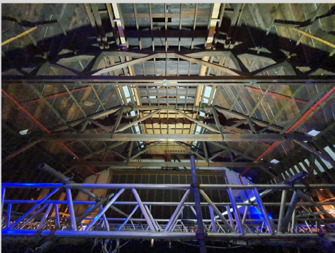
From left to right: Stage house roof structure / Unprotected wiring / Stage house wall timber structure (no lining or insulation) / House curtain rigging / Stage drapes / Fly floor railing & rigging scaffolding
