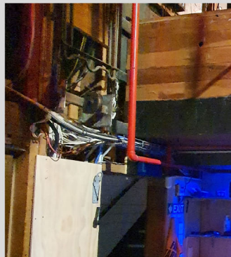
From left to right: Stage house roof structure / Unprotected wiring / Stage house wall timber structure (no lining or insulation) / House curtain rigging / Stage drapes / Fly floor railing & rigging scaffolding
