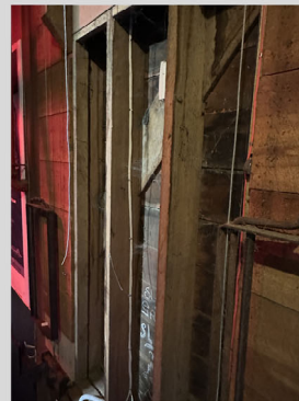
From left to right: Stage house roof structure / Unprotected wiring / Stage house wall timber structure (no lining or insulation) / House curtain rigging / Stage drapes / Fly floor railing & rigging scaffolding
