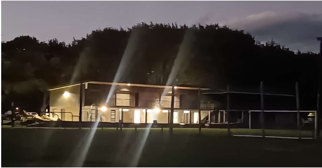
The new Football Centre at twilight
