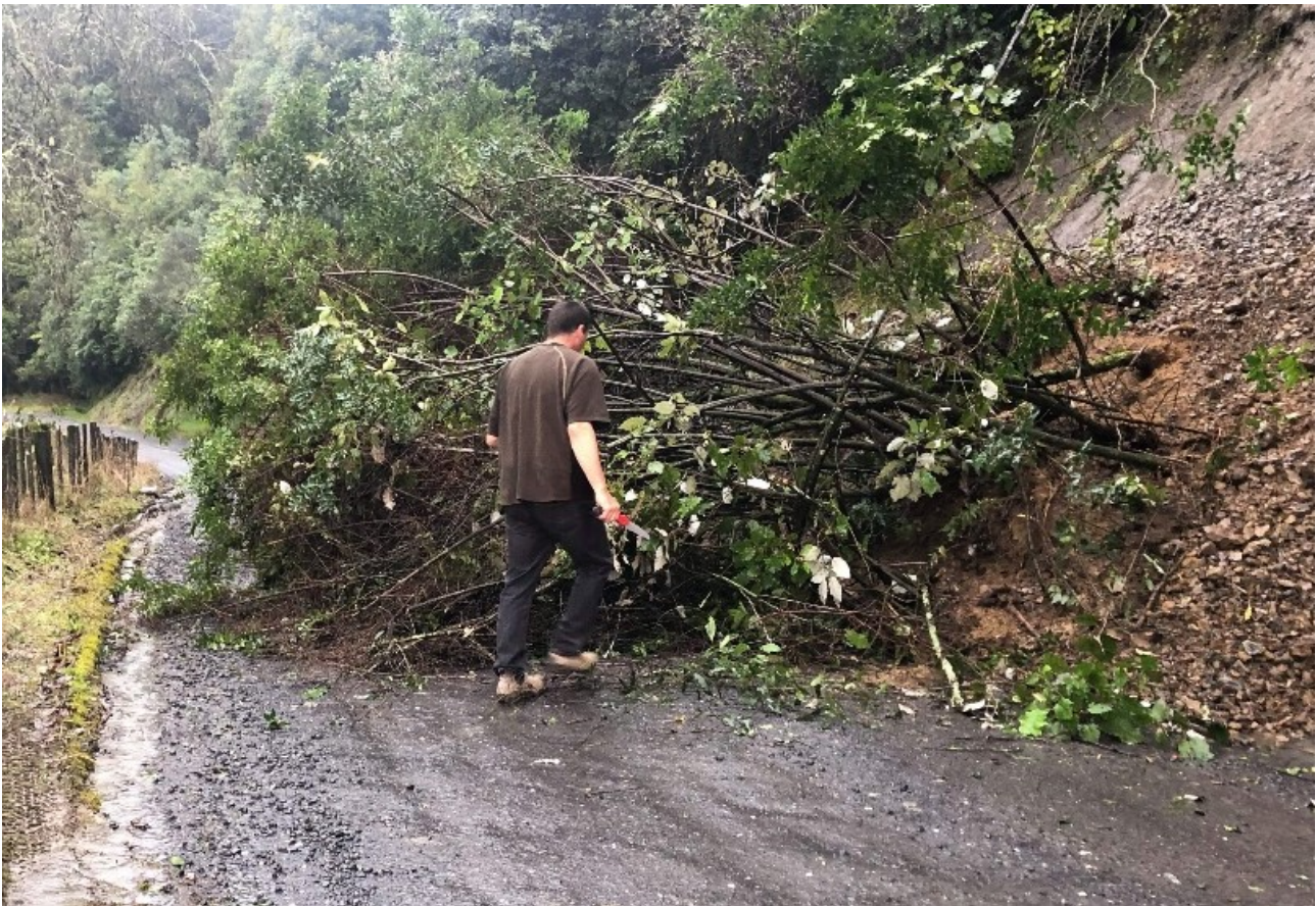
Photo 7: Whanganui River Road small Slip – 5 July 2019. A local trying to clear it.
