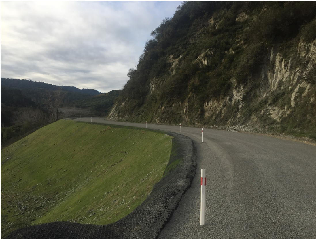
Photo 4: Completed sealed road surface, above Kauwaeroa Dropout site
