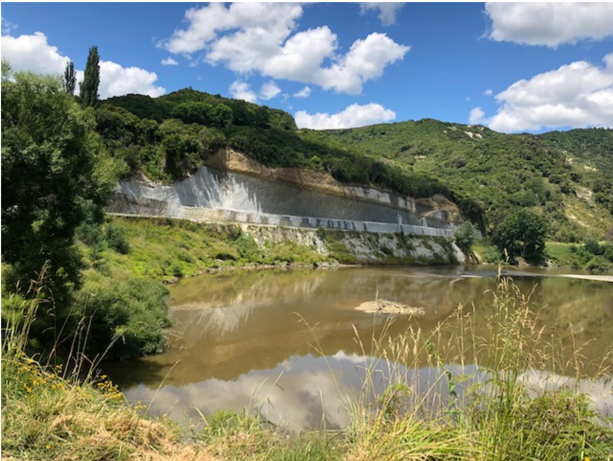
Photo 6: Taken standing on the August 2018 Jerusalem dropout, looking over to the June 2015 completed repair
