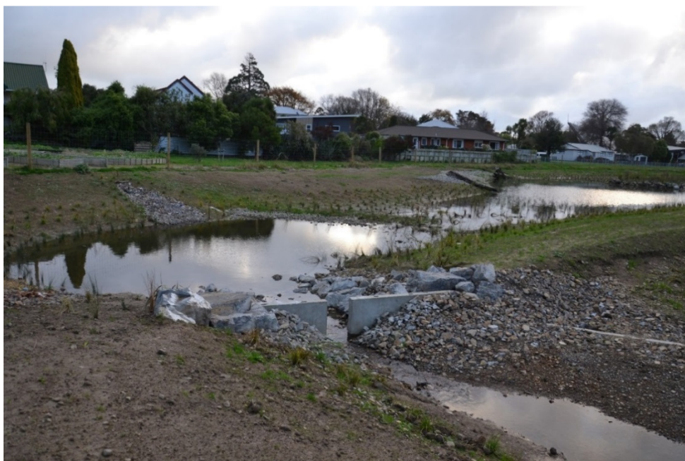
Figure 5. Wetland inlet diversion and bypass, Norton Park, Palmerston North
