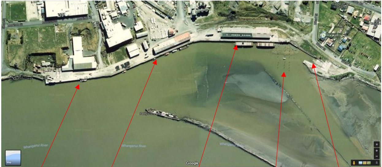
No.1 wharf No.2 wharf No.3 wharf Old piles Boat ramp
