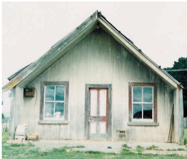
Photo 1: Te Aputa Ki Wairau before it was demolished in 1986. Source: Family collection held by Mihi Davis.
